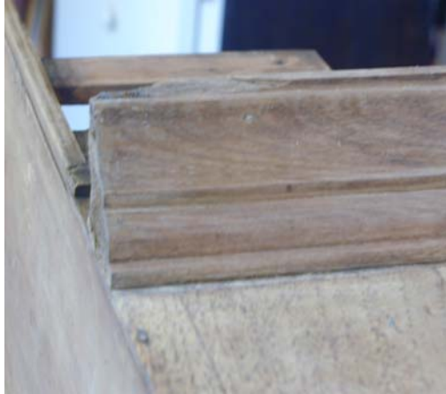
Broken molding
