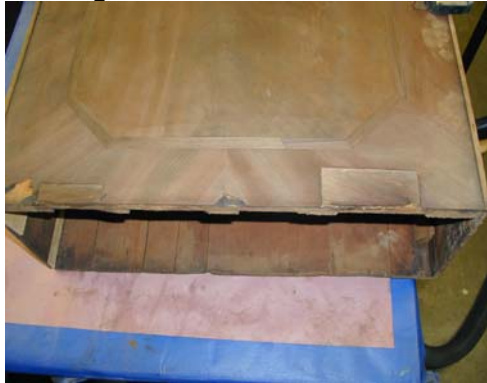
Damaged Case Veneer
