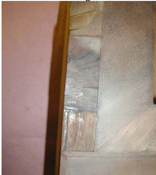
Side Veneer Damage
