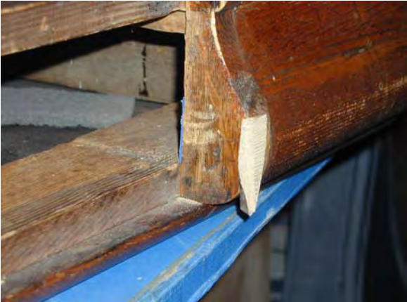
New White Oak scarf joint repair
